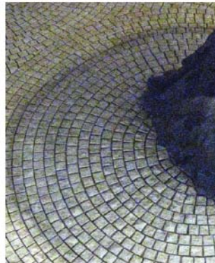
Concentric Circle Paving Granite sets laid in concentric circles
