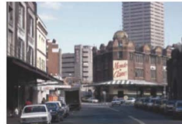
1980 Thomas Street showing axial view to corner tower.
